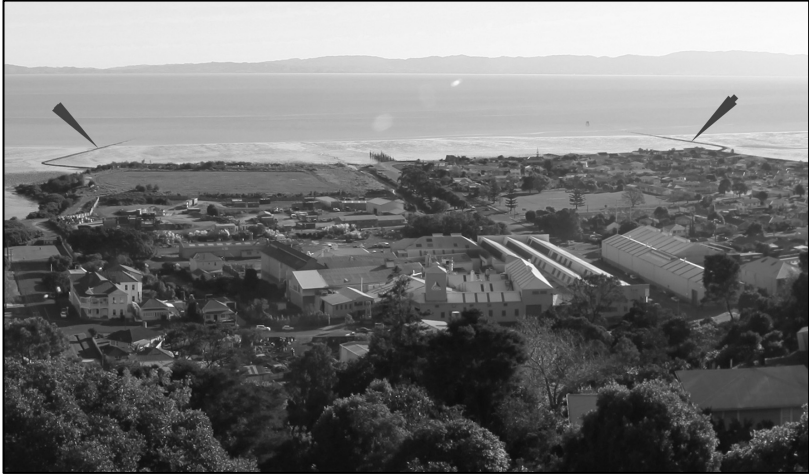
Figure 5. Burke St harbour - lateral breakwater walls indicated (Eric Gosse photo, taken from top of WW1 monument, Waiotahi Valley).
