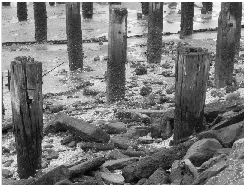
Figure 4. Large timber piles at landward end of the wharf structure; these were probably part of the original 1870s construction.
