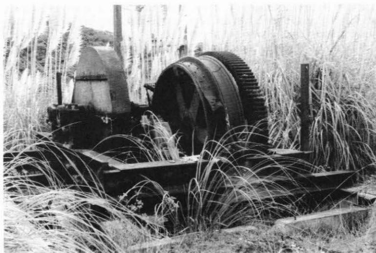
Plate 2. Winding gear and motor, Rotowaro No. 1 mine (S14/149).
