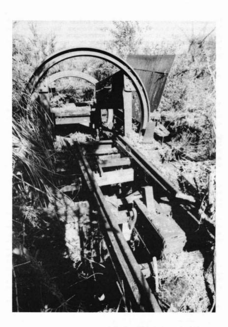
Plate 3. Renown mine rope-road tippler, Rotowaro (S14/152).
