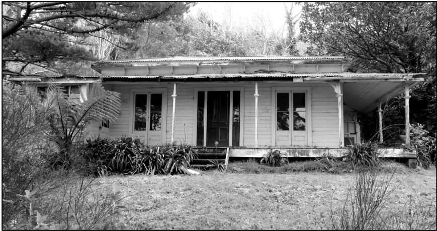
Figure 1. ‘The Wigwam’ prior to demolition, 6 th September 2018.
