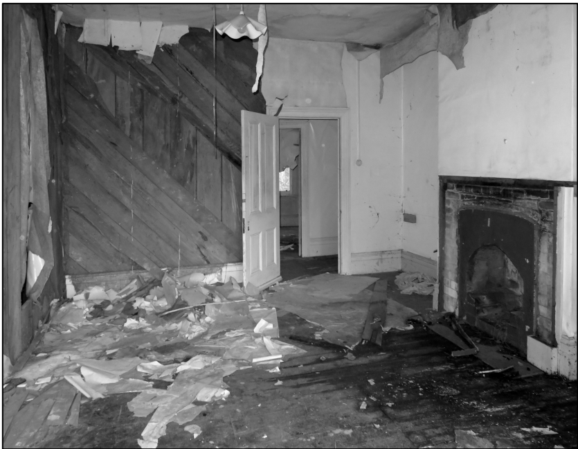
Figure 7. The Wigwam Room 3 (living room) showing structural layers.
