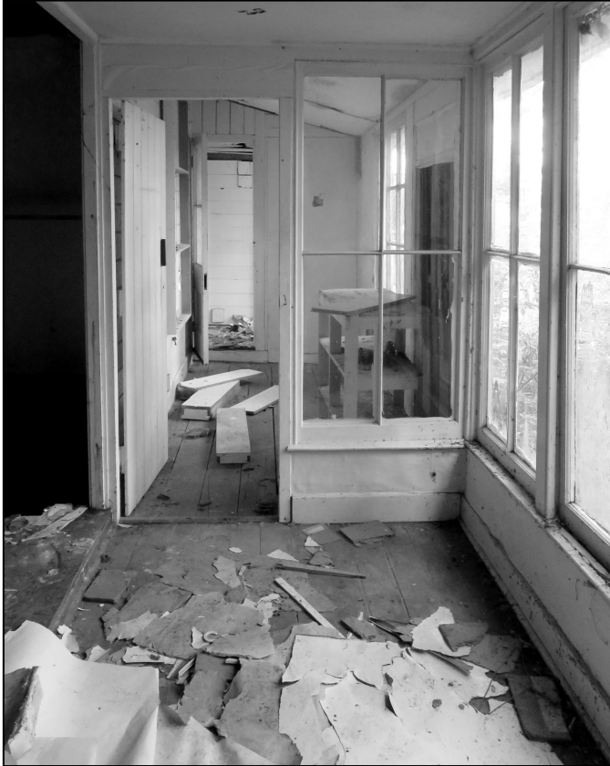
Figure 8. The Wigwam, covered verandah from Room 3a facing south-east.
