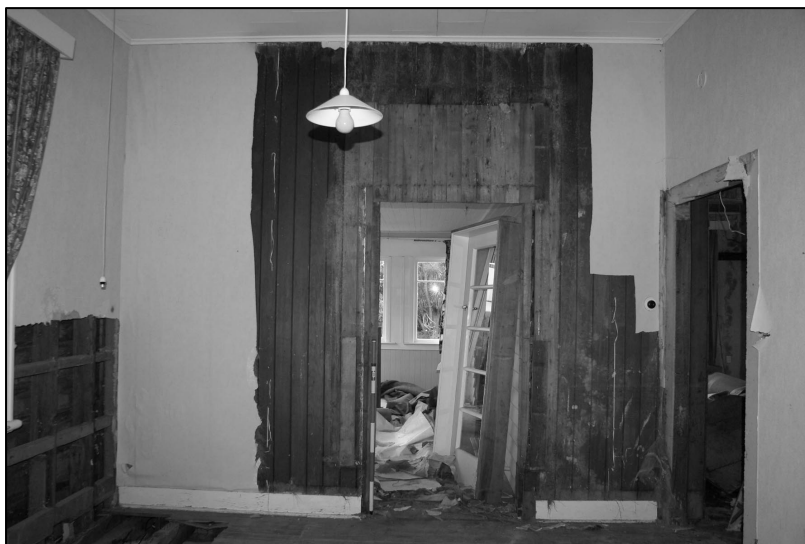
Figure 9 (below). Varnished match lining in what was originally the kitchen. The outline of a former south-east window removed in the 1927 alterations is also visible.
