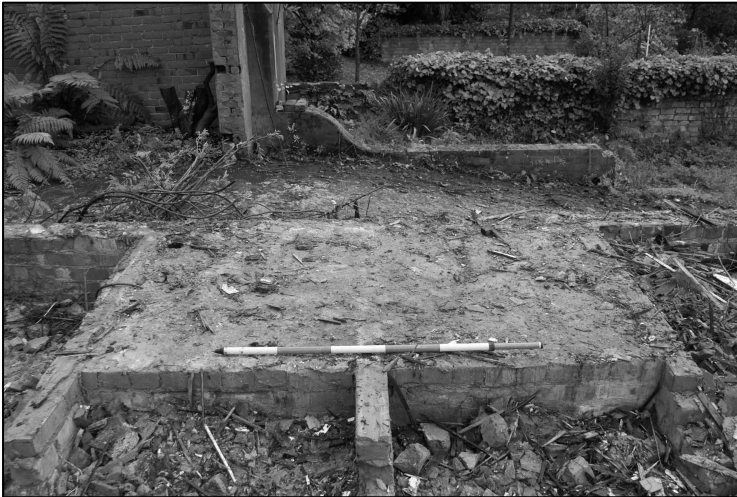
Figure 10. Original kitchen range foundation visible after the building demolition.
