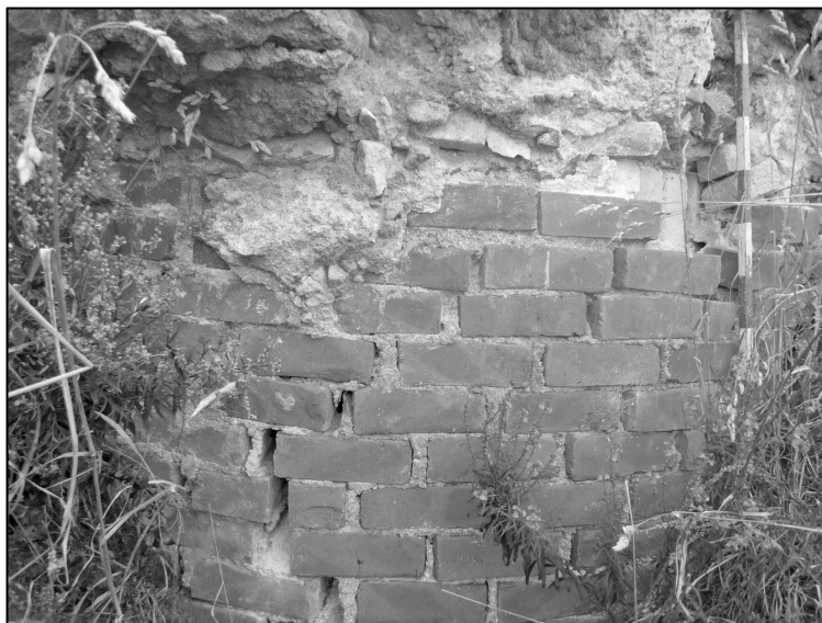
Figure 7. Brick repair in the Fortification Road limekiln.
