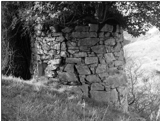
Figure 1. The first limekiln at Sandymount on the Otago Peninsula (site I44/85).
