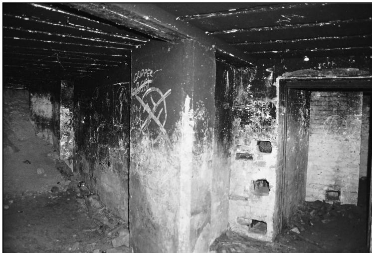
Inside the Kau Point Battery casemate and ammunition store in 1997 (Peter Cooke).
