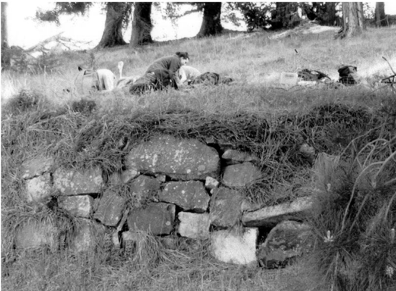
Figure 2. Drystone wall on the down-slope side of the hut terrace, looking west.
