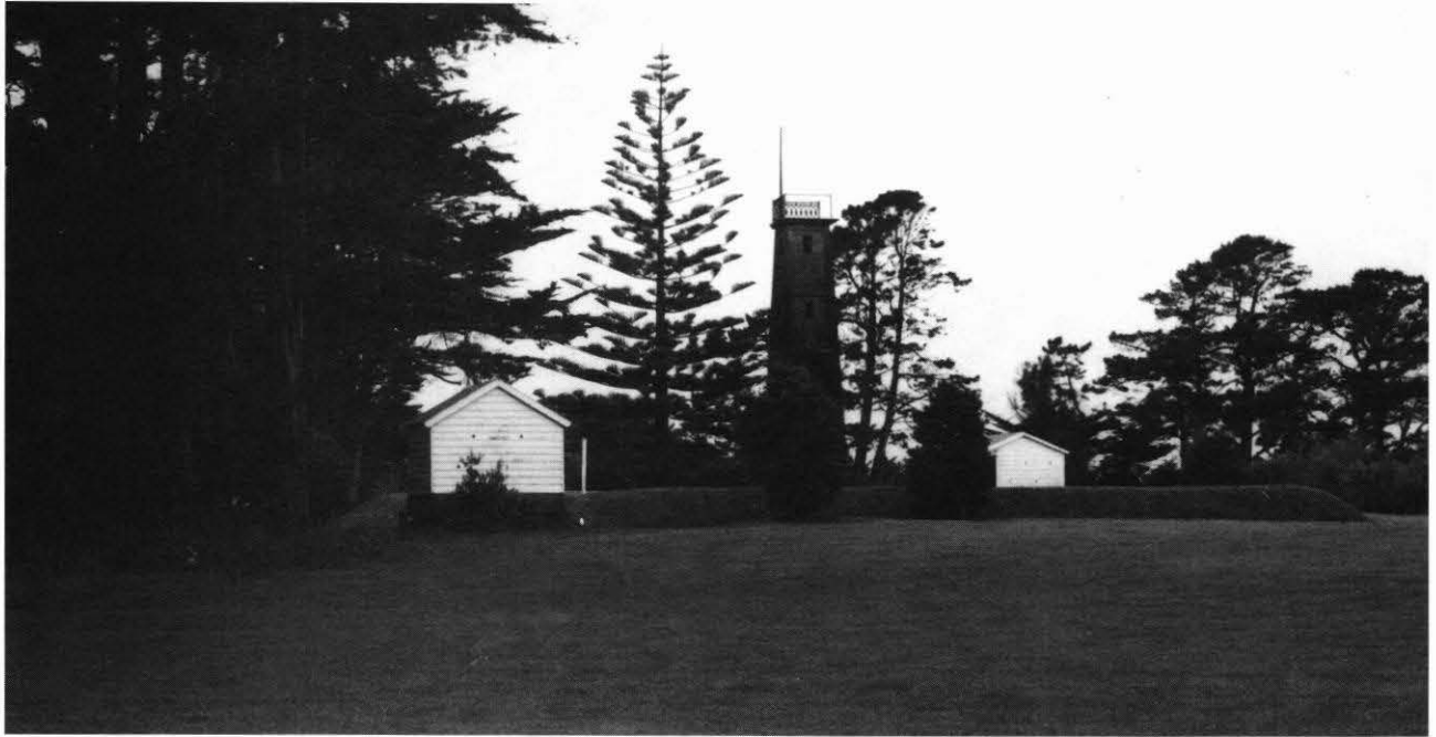
FIGURE 1.10. Manaia Redoubt, 1880. Two loop-holed single storey blockhouses at opposite corners serve as bastions for an earthwork redoubt. Excavation was to reveal a similar blockhouse at the north-west angle of the second (1867) redoubt at Warea.
