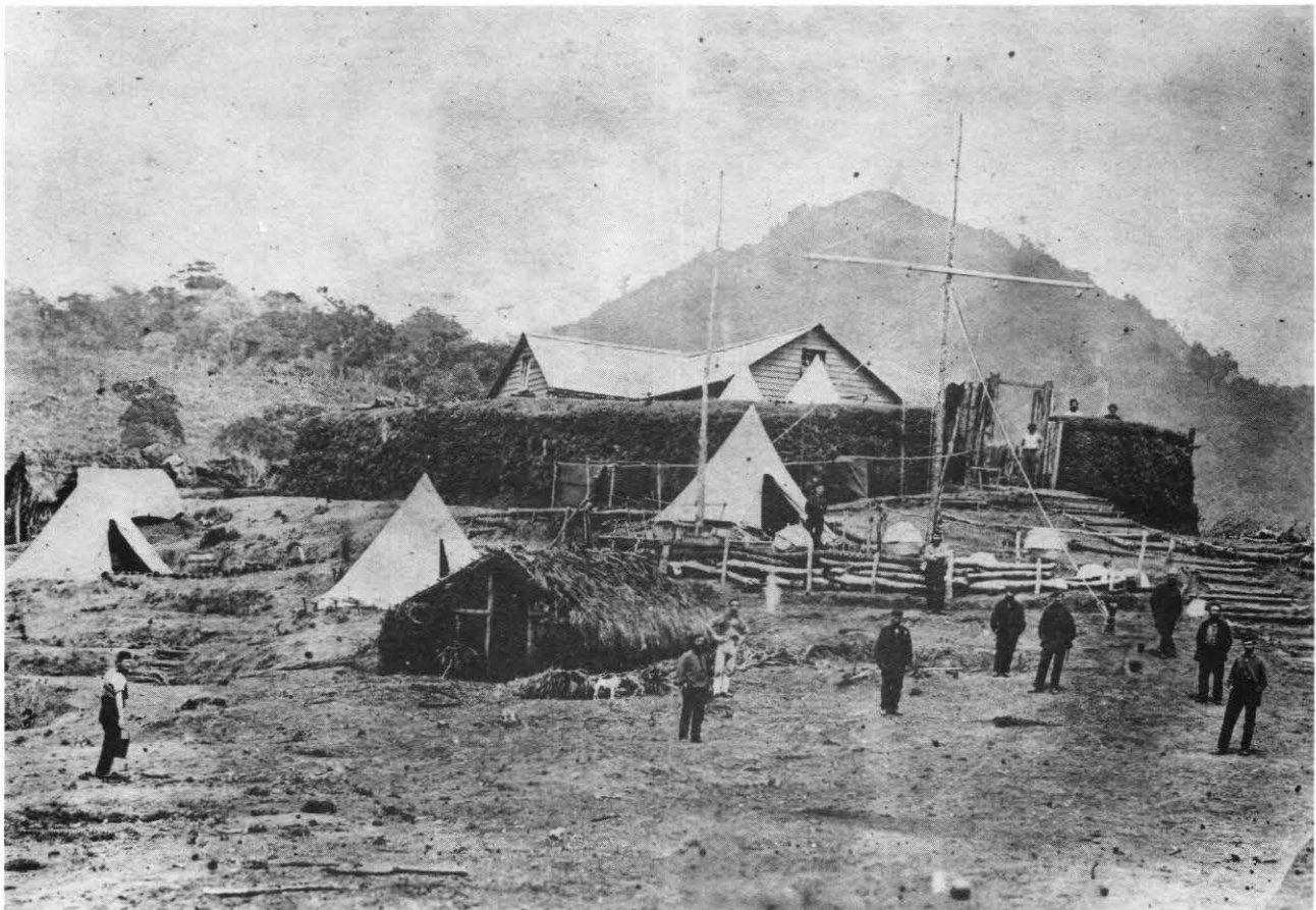
FIGURE 1.6. Kaitake Redoubt, 1864, showing earth and fern construction of redoubt wall, a barrack building ('blockhouse') inside, and outside, a signal mast, bell tents and thatched hut dug into the hill slope. (Alexander Turnbull Library, Wellington.)
