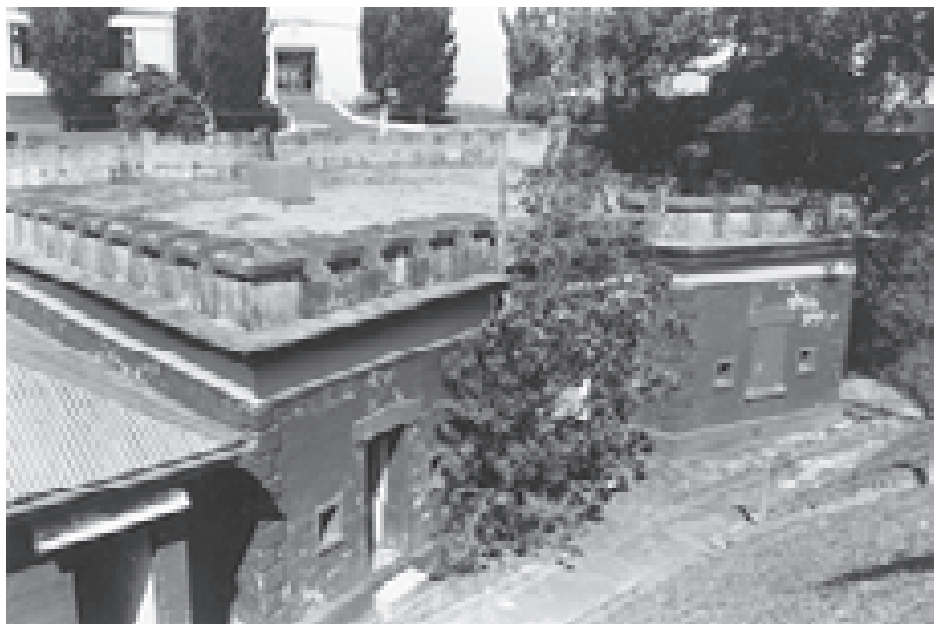
Figure 31. Castellated, demi-bastioned barrack building behind the guns of Fort Takapuna, Auckland, late 1880s (N. Prickett).
