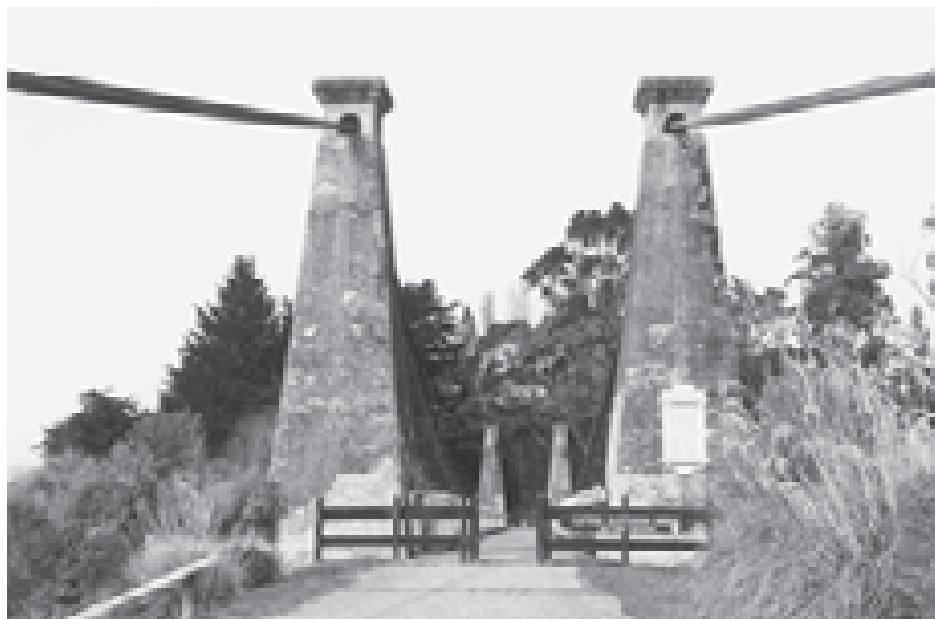
Figure 32. The 1899 Clifden suspension bridge, western Southland (N. Prickett).
