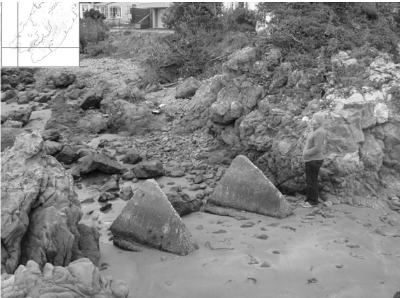
Figure 14: Worser Bay tank obstacles [1942] (R27/256)
