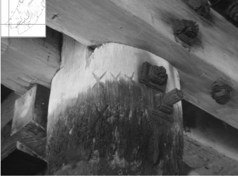
Figure 11: Waterloo Quay wharf [1882]. Assembly marks on original piles
