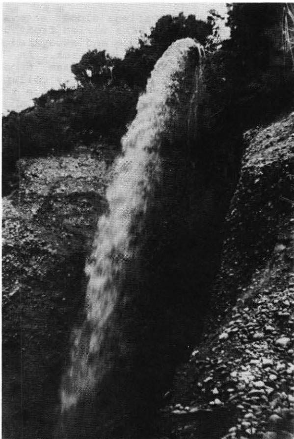
Figure 2. Ground sluicing on the western face of Sulky Gully in 1937. This method of extracting gold from alluvium involved passing a stream of water over the face of a terrace to assist with the mobilisation of gravels by pick, bar and rake. It is a laborious, but simple and inexpensive way of putting increased amounts of material through a sluice-box.
