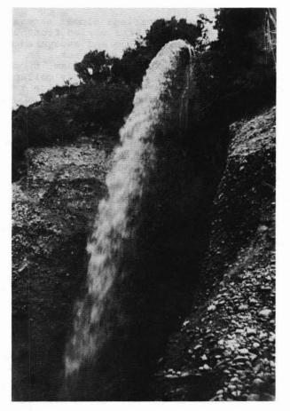
Figure 2. Ground sluicing on the western face of Sulky Gully in 1937. This method of extracting gold from alluvium involved passing a stream of water over the face of a terrace to assist with the mobilisation of gravels by pick, bar and rake. It is a laborious, but simple and inexpensive way of putting increased amounts of material through a sluice-box.
