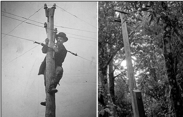
Figure 8. **Left:** Final stages of cable installation on a pole; in this case, carrying multiple lines. This is probably a telephone installation, as telegraph wires that close would interfere with each other, at a high DC voltage. (Te Papa on-line digital image collection) **Right:** Restored telegraph pole on the Old Wires Track
