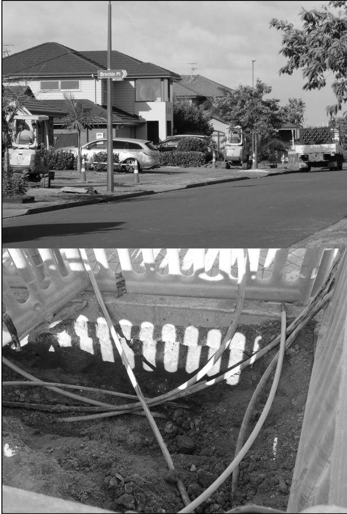
*Figure 9. Although laying a fibre infrastructure underground tends to avoid visible environmental effects (top), it leads to a congested sub-surface (bottom) with attendant maintenance difficulties, and problems with future upgrades. (This is currently being experienced in many cities, with underground water and sewage reticulation requiring urgent replacement.)*
