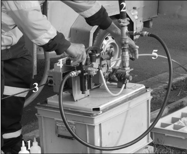
Figure 7. Individual (or multiple) fibres are installed in the ducts by 'blowing.' When ducts are installed, they are constructed to be air-tight. Lubricating gel is inserted from one end (1). A compressor on the back of the truck (2) raises an over-pressure in the duct. The fibre component (3) is fed between
