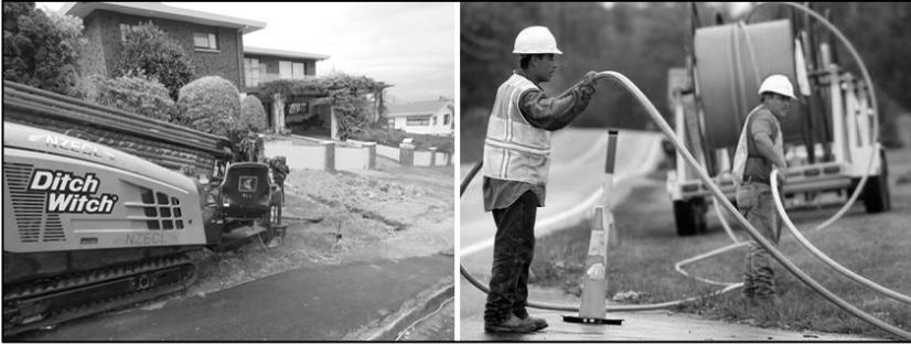
Figure 2. **Left:** Thrusting. **Right:** Drawing duct back through thrust tunnel
