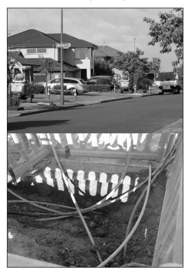
Figure 9. Although laying a fibre infrastructure underground tends to avoid visible environmental effects (top), it leads to a congested sub-surface (bottom) with attendant maintenance difficulties, and problems with future upgrades. (This is currently being experienced in many cities, with underground water and sewage reticulation requiring urgent replacement.)
