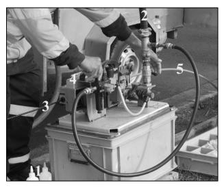
Figure 7. Individual (or multiple) fibres are installed in the ducts by 'blowing.' When ducts are installed, they are constructed be air-tight. Lubricating gel is inserted from one end(1).Α compressor on the back of the truck (2) raises an overpressure in the duct. The fibre component (3) is fed between
