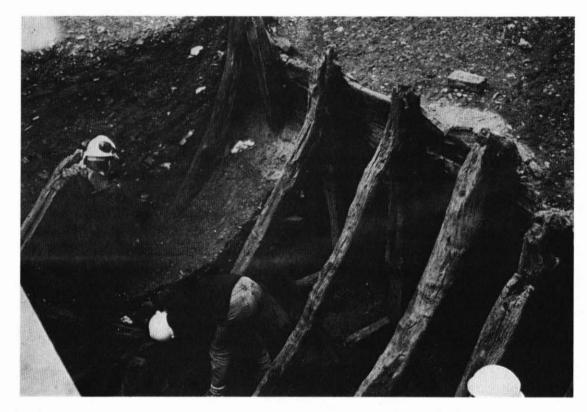
Figure 1. Front braced thirteenth century revetment. Note the buildup of foreshore rising up against the front of the revetment and later dumping on top of that.
