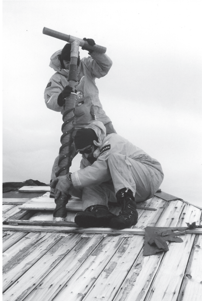
Figure 7: Geoff Ashley and Ted Bugg using a Spire corer to determine snow accumulation within the workroom roof at Mawson's huts, 1997–98 (courtesy of Alasdair McGregor, Australia).
