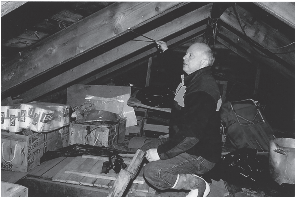
Figure 10: Fred Goldberg documents the roof of Nordenskjöld's hut on Snow Hill Island, 2000–01 (courtesy of Fred Goldberg, Sweden).
