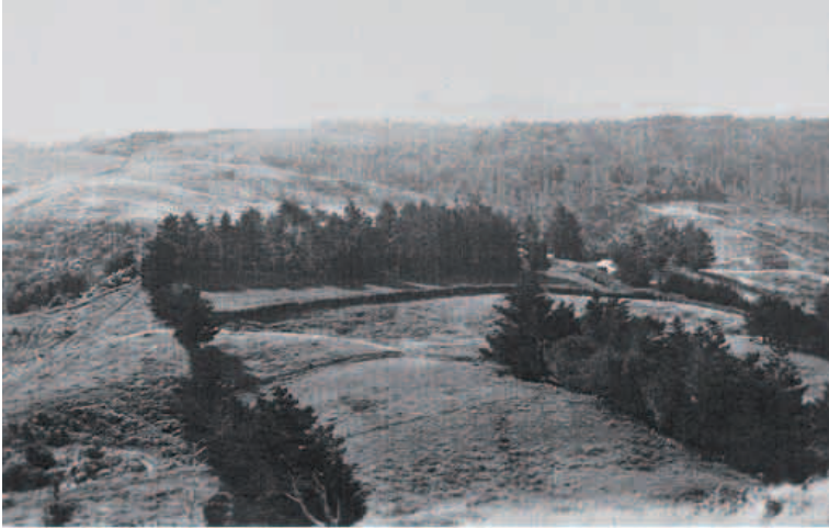
Figure 7. View of The Pines area from the memorial lookout hill in the 1920s, with Maunaupaki (Camel's Back) on the horizon. The light-coloured building in the middle ground is the stable built by the Lyes family. The homestead was behind the large pine tree immediately to the left of the stable.
