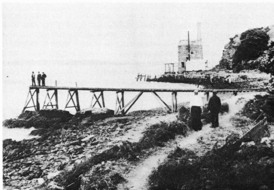
Figure 21: The wharf at Copper Mine Bay, with remains of the 1840s engine house in the background. The small shed in front of the latter houses the engine used to dewater the mine c. 1900. Auckland Institute and Museum photograph, C23047.
