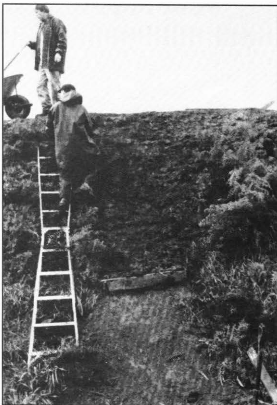
Figure 4. The upper part of the same rut after the rotten turf has been hand-tamped and a smooth surface created for overlying the instant turf.
