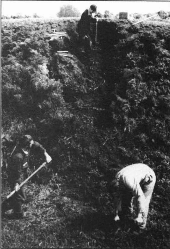
Figure 2. View showing initial backfilling of the rut on the west wall of the Alexandra redoubt using displaced material. All the ruts were created by children sliding down the slopes.
