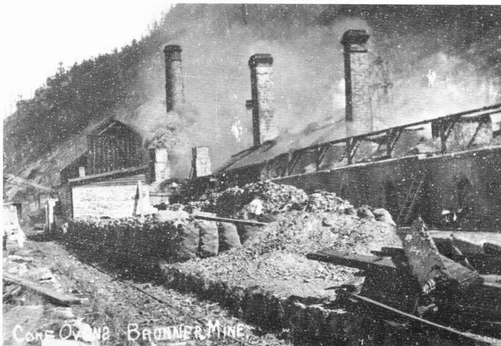
BRUNNER Plate 2. Ovens and bagging platform early 1900s, showing stone retaining wall. Chimney at right services the ovens.
