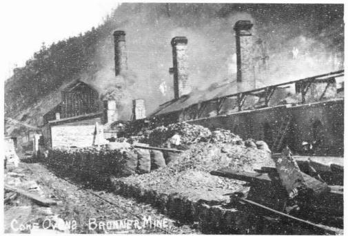
BRUNNER Plate 2. Ovens and bagging platform early 1900s, showing stone retaining wall. Chimney at right services the ovens.
