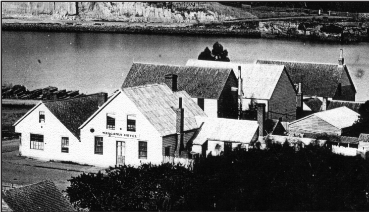
Figure 6. The Wanganui Hotel in the 1870s showing the three adjoining buildings with annexe out the back (National Library Ref. No. 222).
