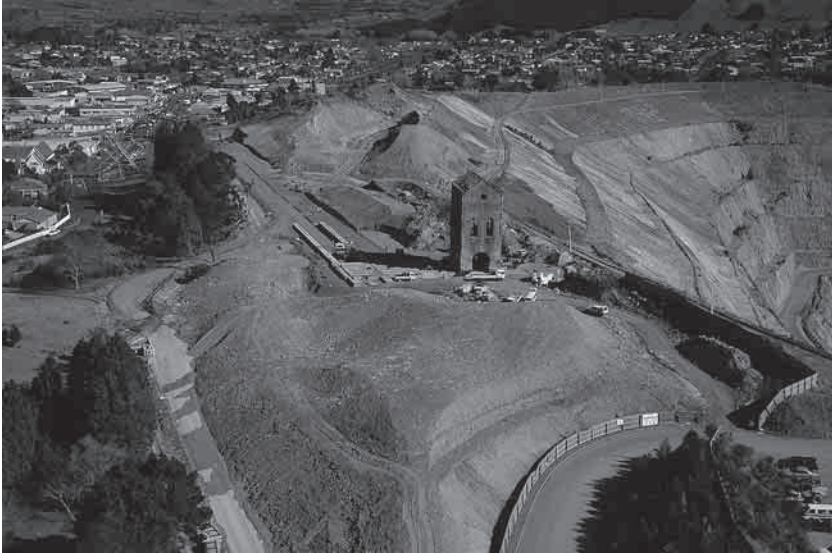
The Cornish pumphouse on the move. Photo Newmont Waihi Gold.
