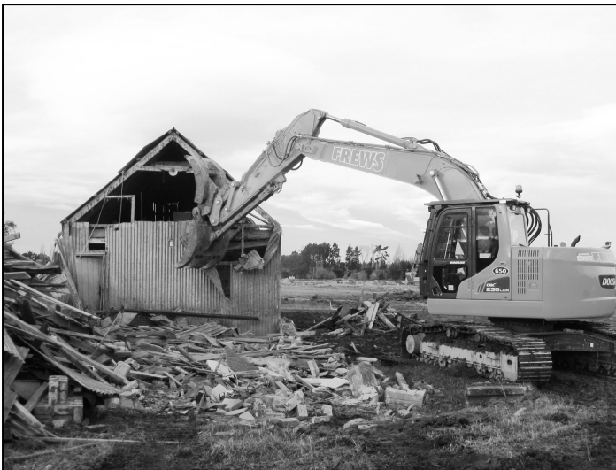
Stripping the iron off an early barn at Woodend (Kevin Jones).
