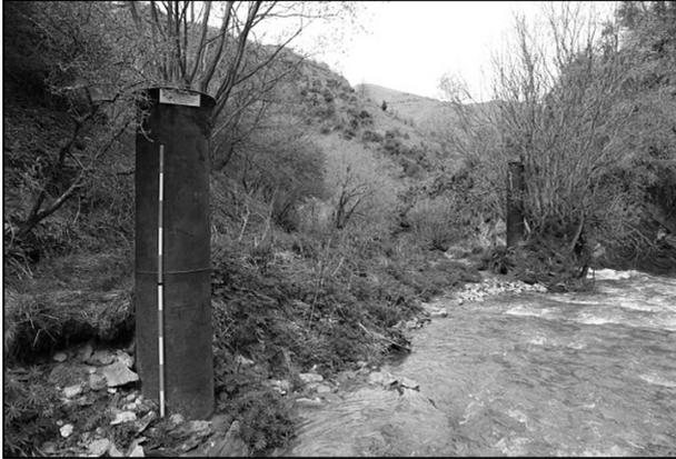
*Old water pipes that were used as piers for a footbridge across Skippers Creek to provide access to the Nugget workings (Matt Sole).*
