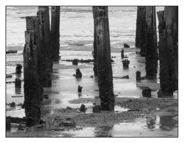
Burke St wharf, showing the stumps of 1870s timber piles between 1920s concrete piles (Dave Wilton).
