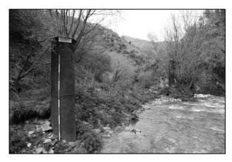
Old water pipes that were used as piers for a footbridge across Skippers Creek to provide access to the Nugget workings (Matt Sole).
