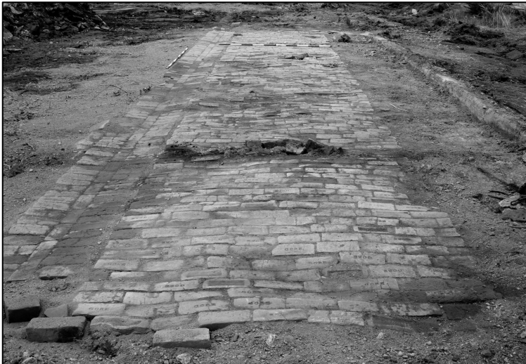
Top: the old barns at Rosebank Farm, Mosgiel. Bottom: Brick floor after barn demolition (both Andrea Farminer).
