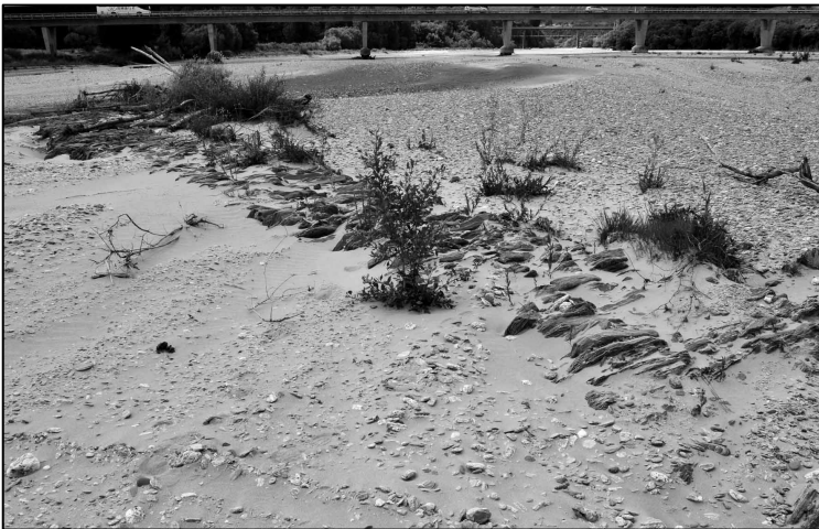
The wing dam that was built to protect the first Shotover Bridge (Ben Teele).
