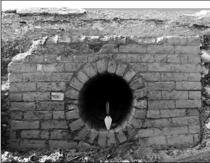
An 1887 brick culvert in Rangiora (Michael Trotter).
