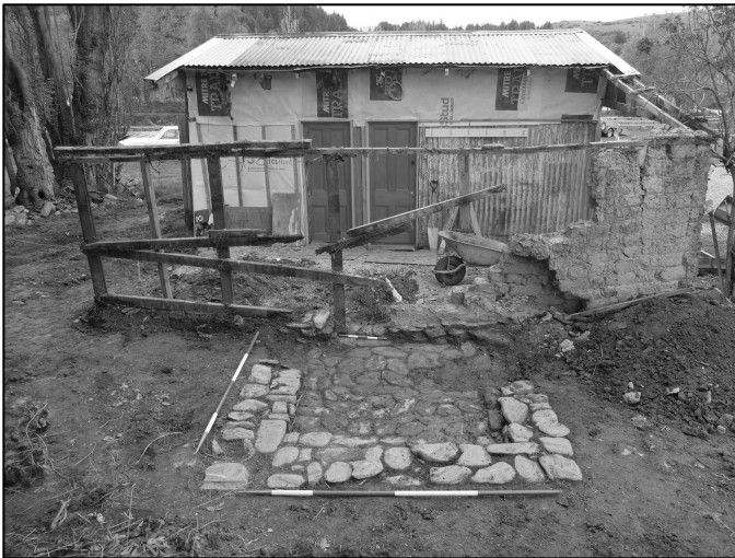
The stone foundations for the rear part of an old mudbrick cottage at Cambrians in Central Otago.
