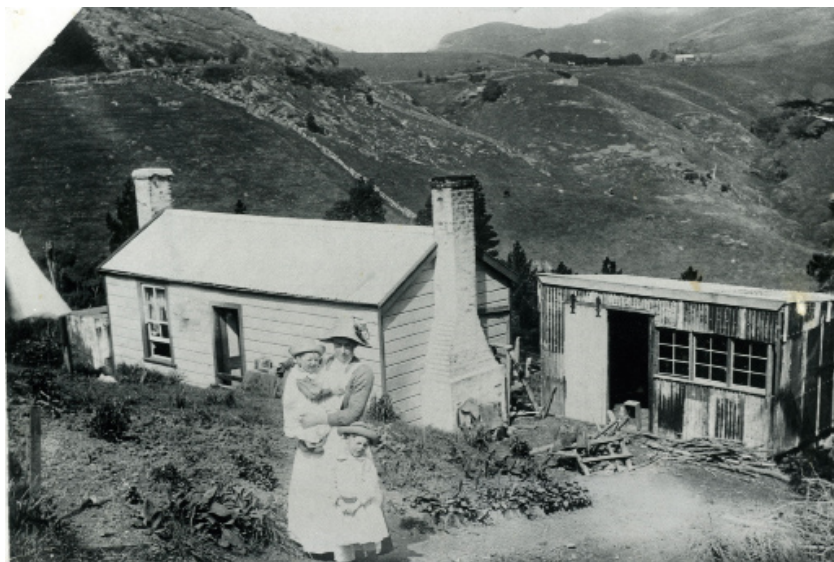
Figure 4. Captain William Leslie's house (I44/82), also the site of the Harbour Cone Cheese Factory. Photograph is dated 1913, showing later occupants. Otago Peninsula Museum.
