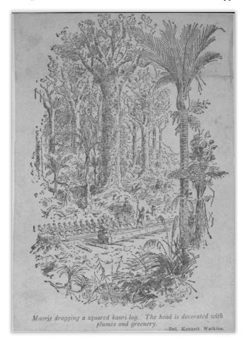
Figure 9: Sketch of Māori contractors hauling a kauri log from the bush at Waiheke Island. Note the 'skidded road' on which the log is hauled. (Webster, Kenneth Athol, 1906-1967. [Clarke, Cuthbert Charles] 18-18 :Maoris (sic) dragging a squared kauri log. The head is decorated with plumes and greenery. Del. Kennett Watkins. [ca 1920?]. Ref: A-111-100. Alexander Turnbull Library, Wellington, New Zealand. <u>http://natlib.govt.nz/records/22816173</u>)
