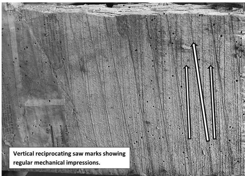
Figure 18. Regular vertical and diagonal marks from a reciprocating saw. Kahikatea wall board from a Lyttelton cottage, c.1853.
