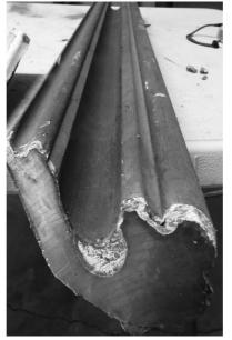
*Figure 20. Kauri scotia or cornice moulding probably made with several different cutters, c.1890.*
