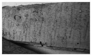
Figure 14. Random marks from a large two-man pit-saw c.1853.
