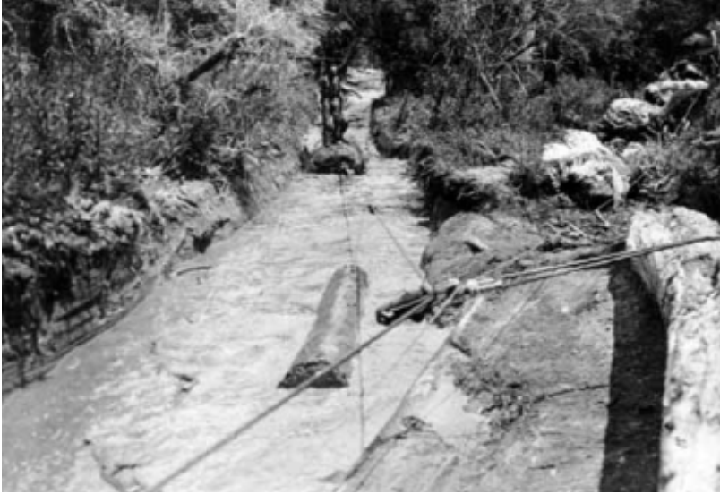
Figure 5: Logs being hauled in a canal, from the Main Booms to the main Kaueranga tramway. Tudor Collins photograph [Archives Reference AAQA 6395 Box 6 M12396] Archives New Zealand The Department of Internal Affairs Te Tari Taiwhenua
