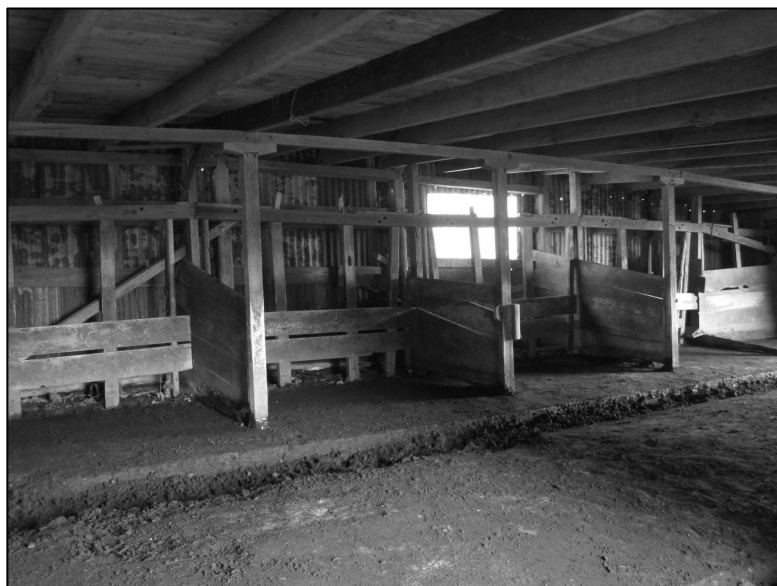
Figure 4. The interior of the byre after the floors were cleared.
