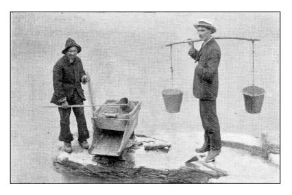
Figure 5. Wing Chung working at his cradle in 1901, with George McNeur of the Presbyterian Church alongside (Don 1923).
