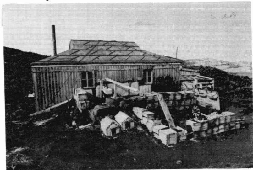
PLATE 2. The NE side of Shackleton's hut (1907-9) at Cape Royds, Ross Island. The structures in the foreground are the remains of the garage and stables which were walled with stacked provision cases.
