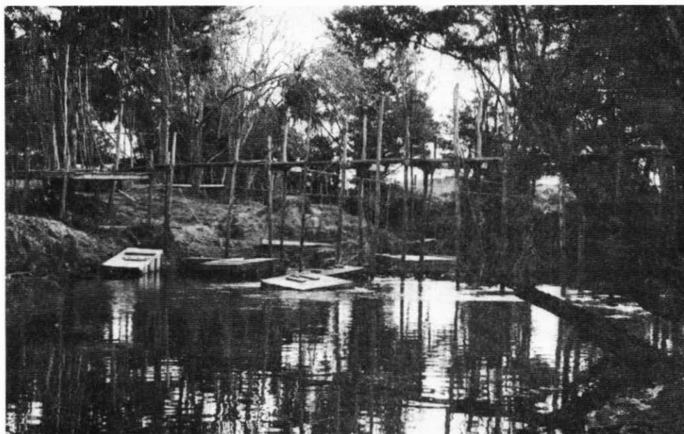
Figure 2: The Baker awa , looking upstream. On the far left is the working platform and in the background is the next awa . Storage boxes can be seen, tied to the awa support poles.
