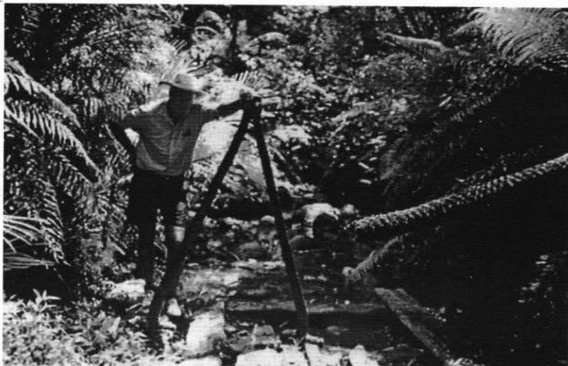
*Jack Diamond in 1975 and an iron wishbone tom, part of the tripping mechanism for the gate of one of the earliest kauri timber dams built in New Zealand, constructed in the Henderson Valley in the 1850s. Photo: Bruce Hayward.*
