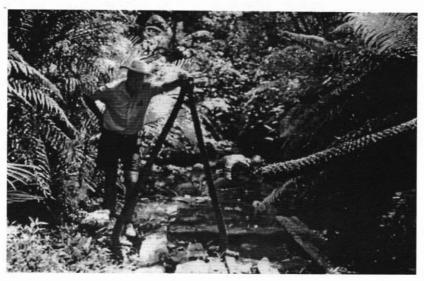
Jack Diamond in 1975 and an iron wishbone tom, part of the tripping mechanism for the gate of one of the earliest kauri timber dams built in New Zealand, constructed in the Henderson Valley in the 1850s. Photo: Bruce Hayward.
