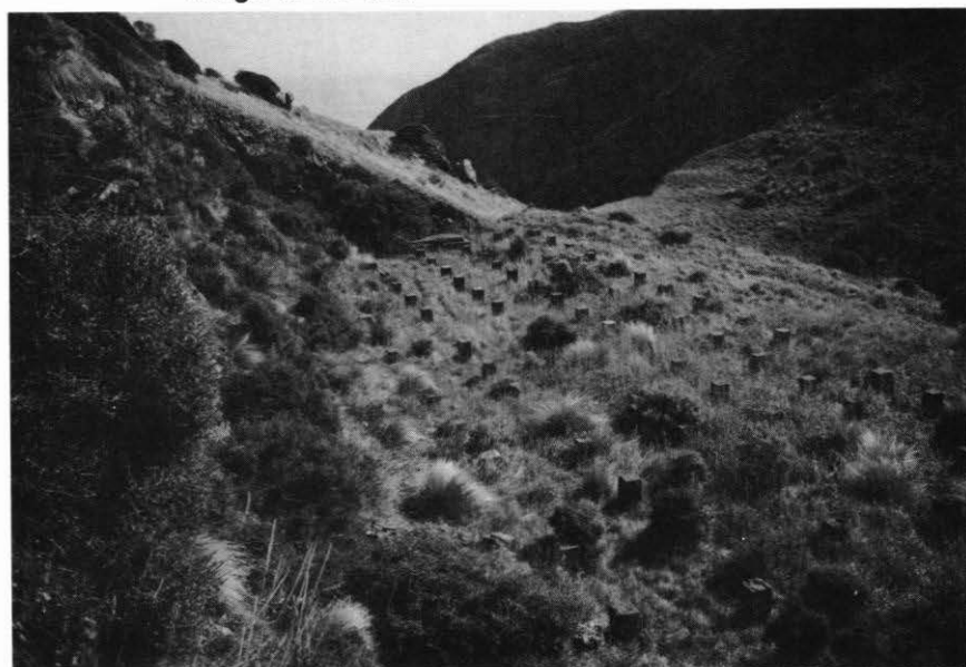
Plate 4. Sinclair Head, 1992. Terrace with concrete piles: remains of the kitchen/living quarters built in 1942.
