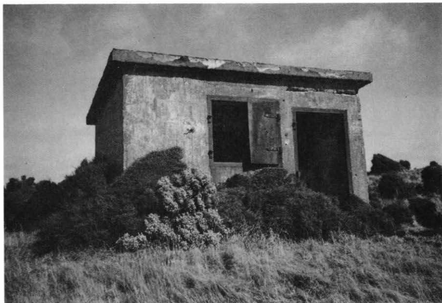
Plate 3. Sinclair Head, 1992. One of the two concrete huts of similar design at the site.
