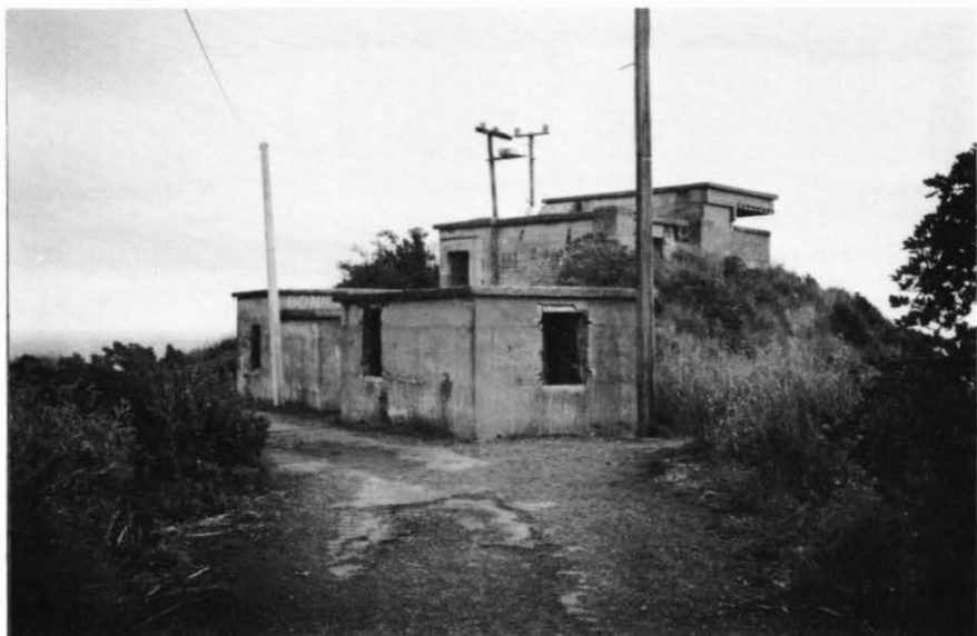
Plate 2. Palmer Head (Moa Point) Radar Station in 1991.
