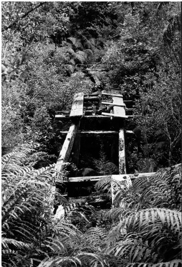
Figure 3. Timber aqueduct over Taylor's Creek.
