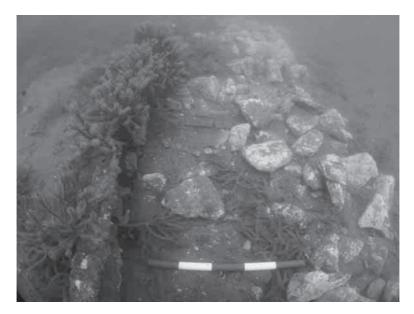
Figure 8. The slipway under water showing roller rail and rock foundation (SCHIP & Subsurface Ltd).
