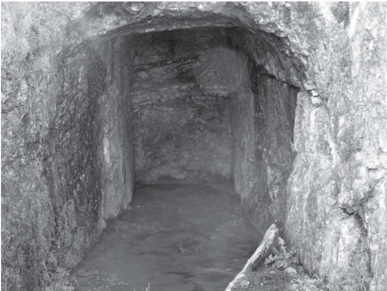
Figure 3. Adit approx. 5 m long.
