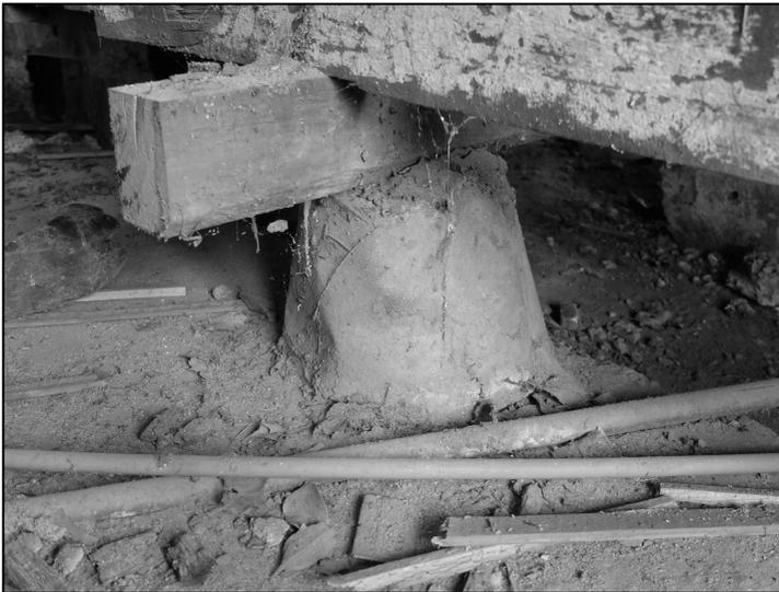
*Figure 7. Bucket shaped concrete pile with the bucket left in place in the 1920 section of the house. These 'bucket' piles were not set into the ground, but just rested on an earlier asphalt surface.*
