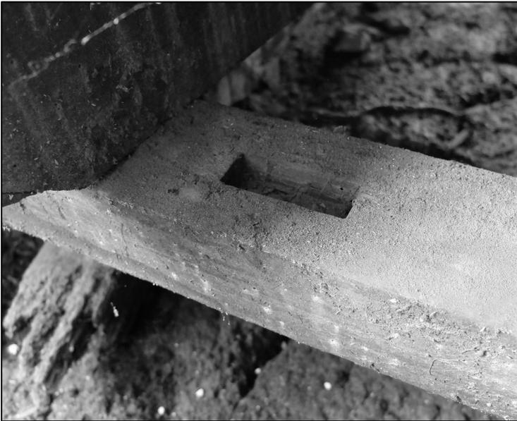
*Figure 8. A floor bearer in the front section of the house with a redundant mortise, evidence of its earlier use, probably as a top or bottom plate of a timber framed wall.*
