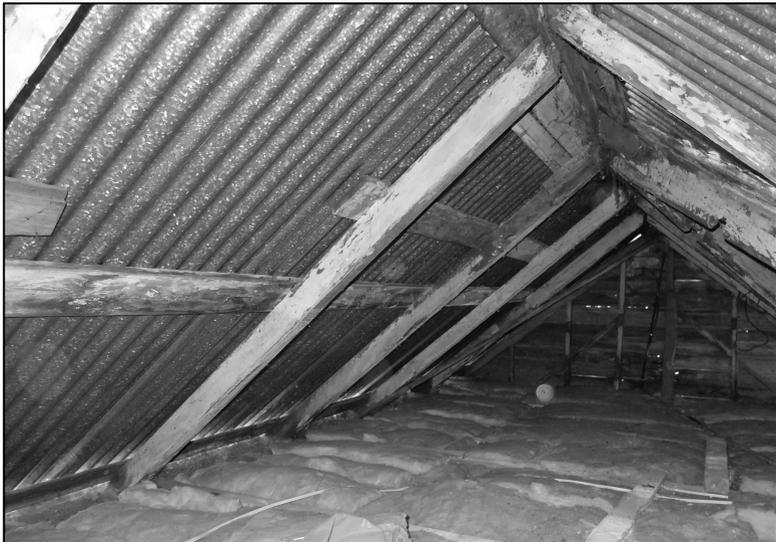
*Figure 9. The very lightweight and sparse framing of the roof at 38 Richmond Street, possible only because corrugated iron was used as the roof cladding.*
