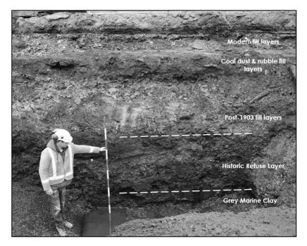
Figure 5. Full section from stormwater pipe section 8 showing the sequence of fill deposits typical across the southern half of the site. Scale is 2 metres high and depth of trench is 3.5m (note: contractor's personnel in picture).
