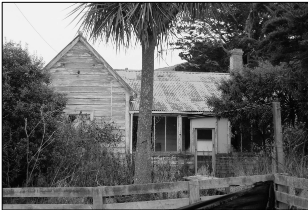
Figure 8. The front of the farmhouse.
