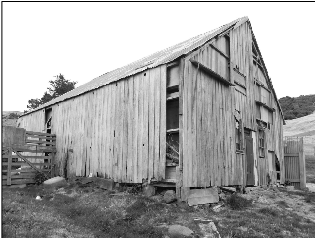
Figure 7. The rear of the cow byre, showing the original board and batten cladding.
