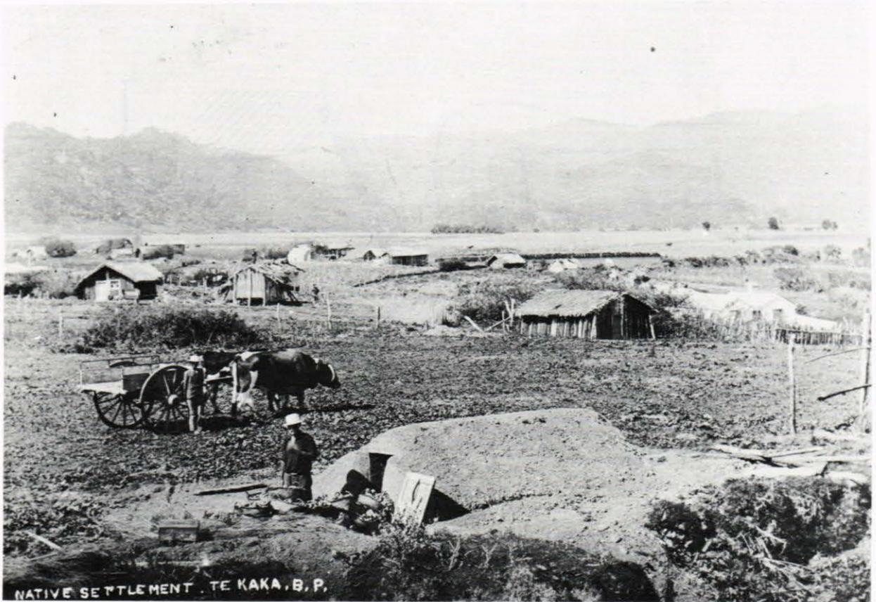
Fig.11 Late 1800's photograph of a Maori settlement at Te Kaha (Te Kaha in photo caption), eastern Bay of Plenty. Kits of kumara are ready for stacking within a newly constructed rua. Thatching is exposed along the base of the roof. (Photo reproduction by Anton van der Wouden, Whakatane Museum)
