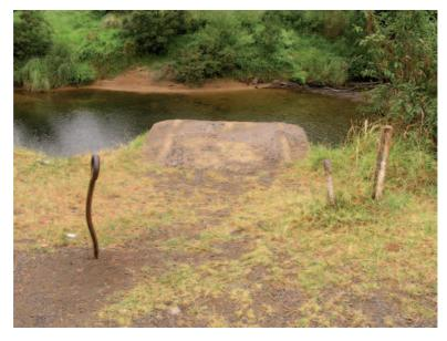
Figure 3. Remains of suspension bridge abutment on northern bank of Kauaeranga River (WP 557).
